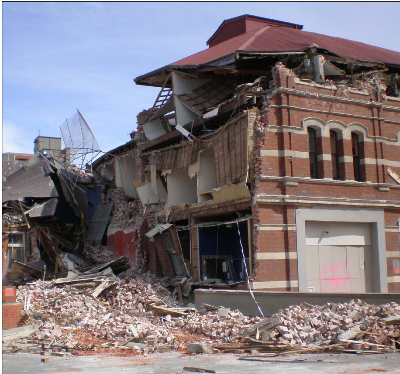
As-built URM building following 22 nd Feb 2011
