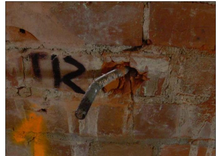
Crushing of brick substrate
