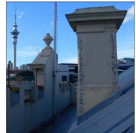
Chimney strengthening
