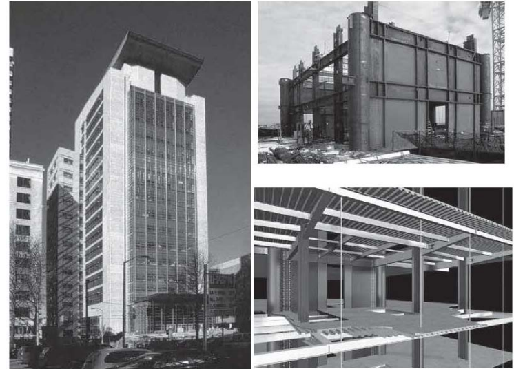
a. U.S. Federal Courthouse, Seattle (20 Steel Design Guide- Steel Plate Shear Wall)
