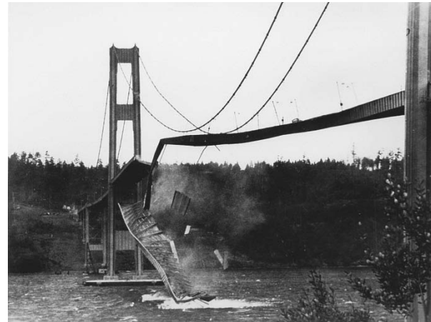
Tacoma Narrows Bridge
