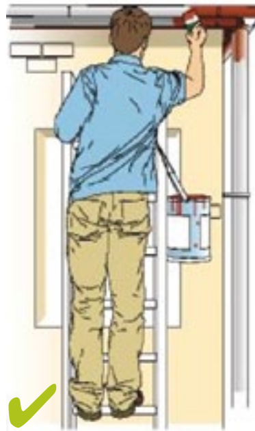
Figure 28: Correct – user maintaining three points of contact with the ladder.
