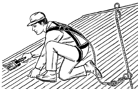
Fig. 4 Appropriate personal protective equipment must be provided and used
