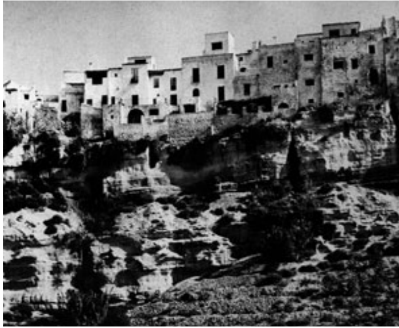
An example of the limited material and colour palettes that increasingly appealed to Athfield. PHOTOGRAPHER NOT KNOWN, AAL ARCHIVE.
