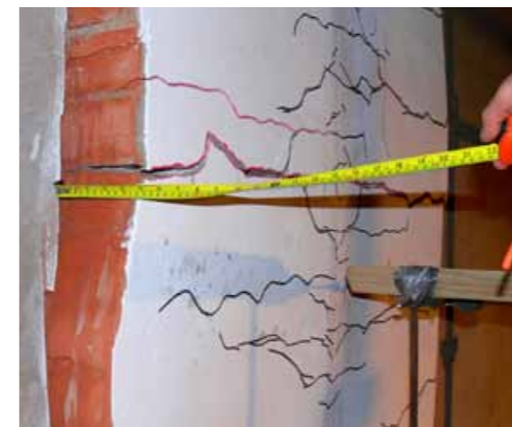
Allen's Trading Complex building, Gisborne, badly damaged in the 2007 earthquake. This image shows crack patterns that developed after implementing and testing a low intervention and low cost technique used to strengthen unreinforced masonry buildings against earthquakes.
