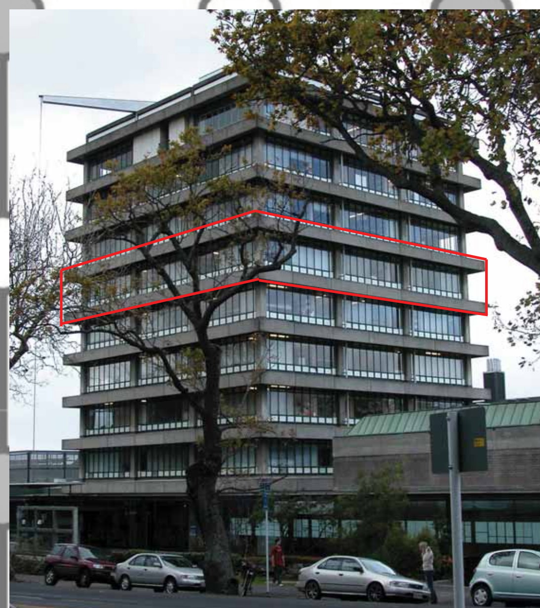
The UoA Engineering Tower is regarded as the most electromagnetically characterized building in the Southern Hemisphere (if not the world).
