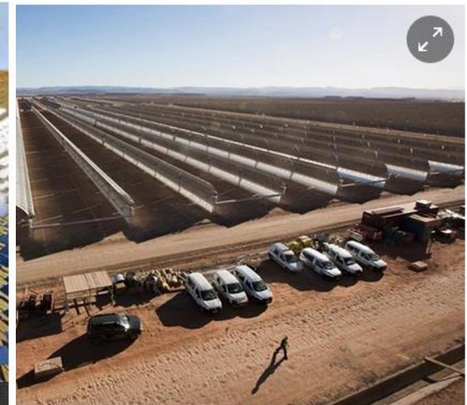
Ouarzazate solar power plant provides 160MW of its ultimate 580MW ion for the Guardian
