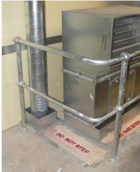
Figure 1: Example of a floor stencil to non-trafficable floor
