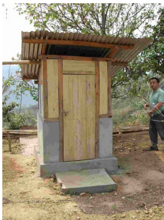
Figure E12 GFF toilet with septic tank behind
